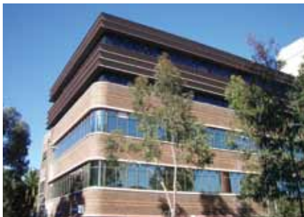
The newly renovated Building 9.
