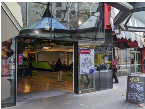
Figure 2. Building 80 North entrance
