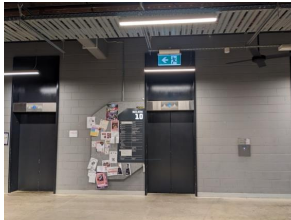
Figure 9. Lift on Building 10
