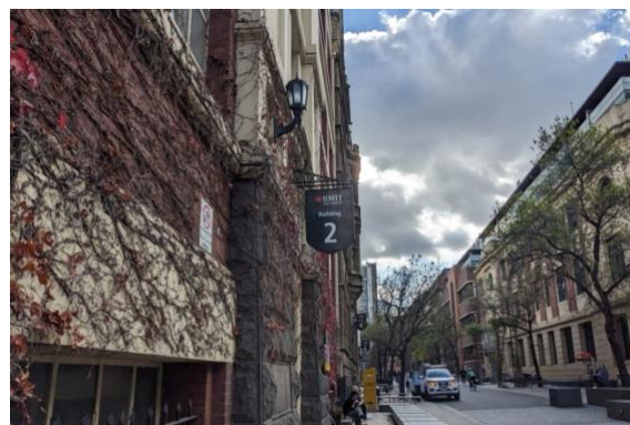
Figure 4. Buildings 2, 4, and 6 on the left side of Bowen Street
